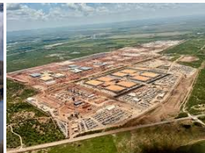
$500B U.S. backed 'Stargate' data center initiative
